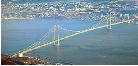
Akashi Suspension Bridge
